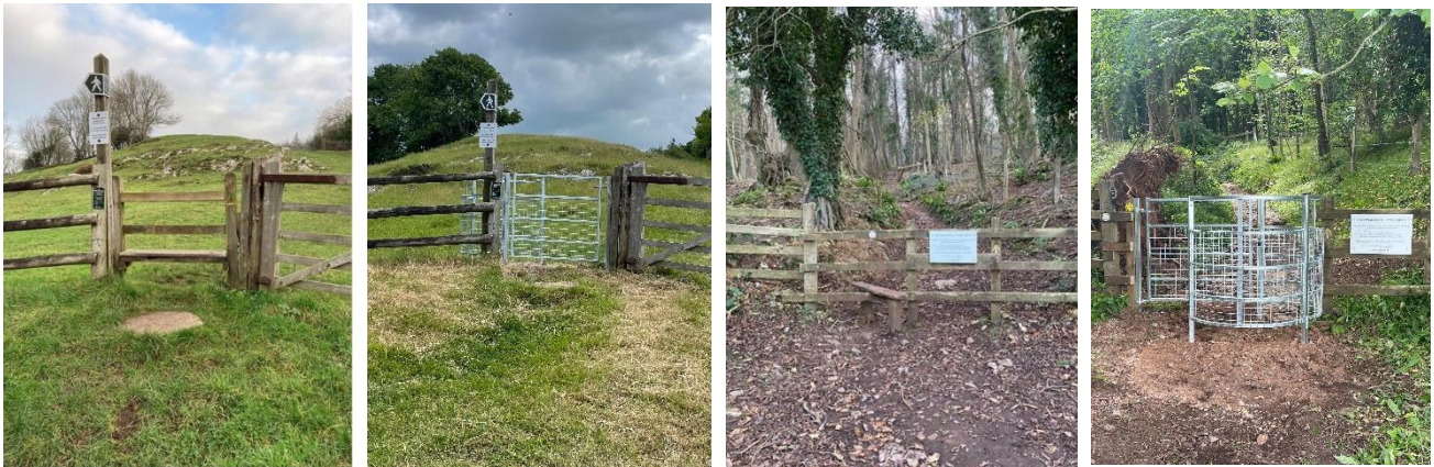
Figure 14 Before and after shots of stile replacements with kissing gates
